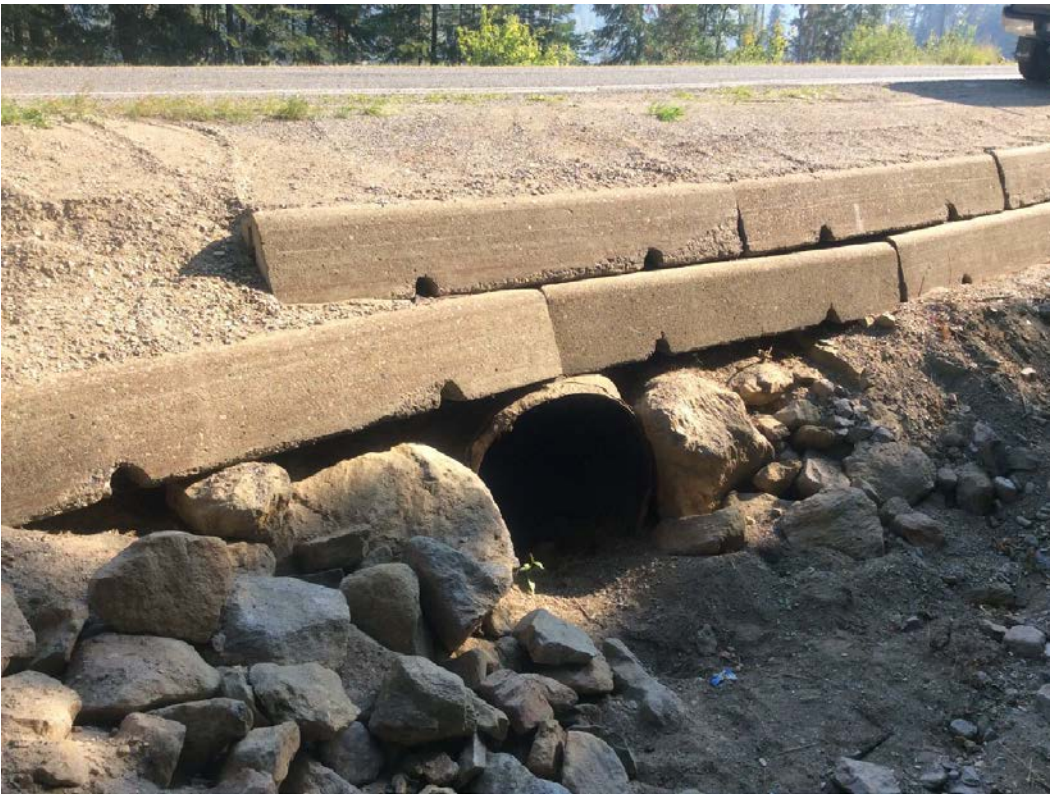
Photo 6: Highway culvert at Unnamed Creek 2.
