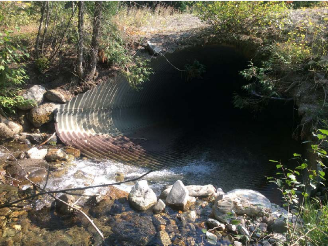
Photo 13: Highway 3 crossing of Topaz Creek.
