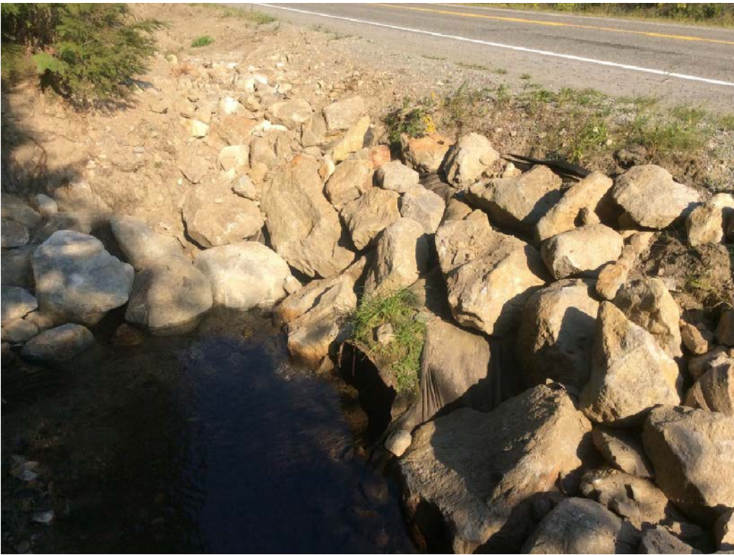
Photo 5: Highway culvert at Unnamed Creek 1.
