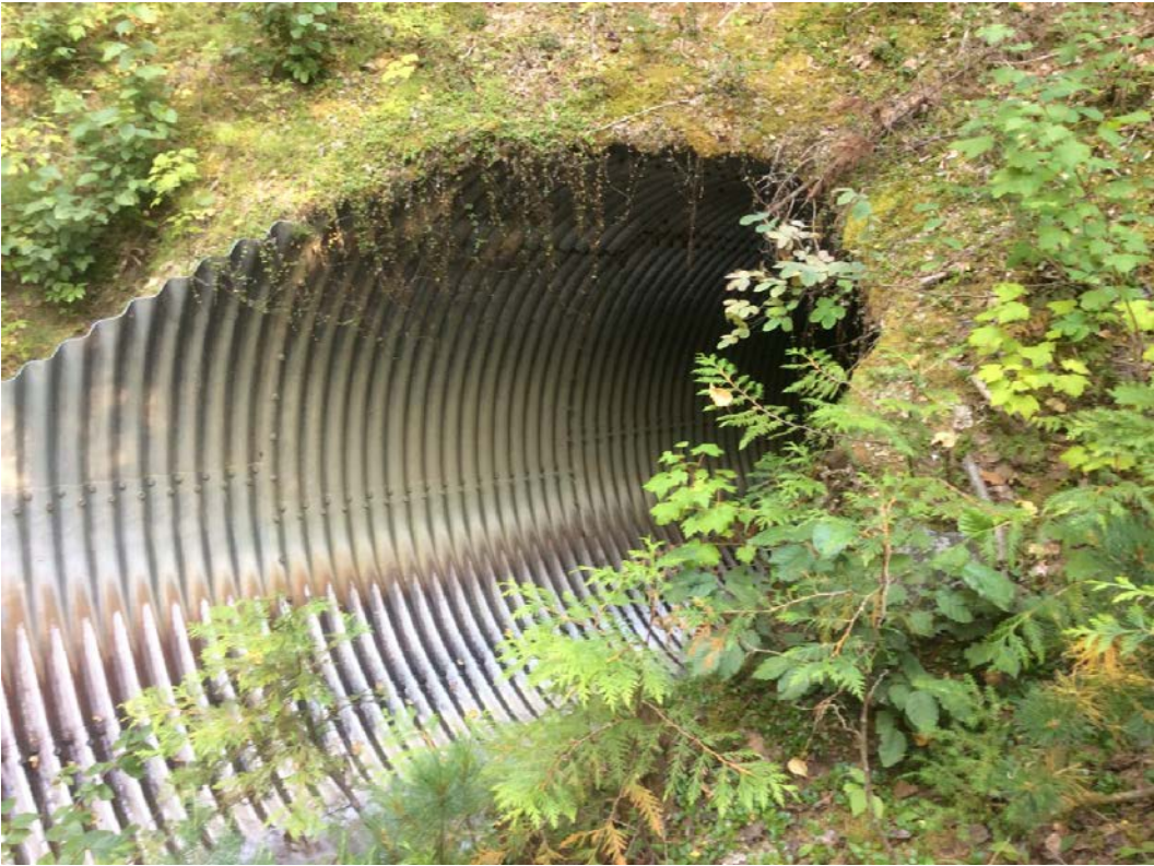
Photo 1: Highway culvert at Placer Creek.
