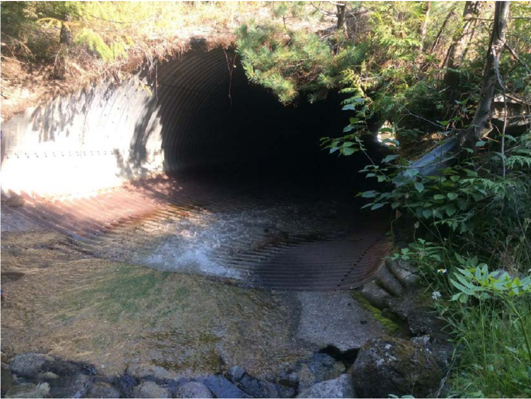
Photo 11: Highway 3 crossing of Toby Creek.
